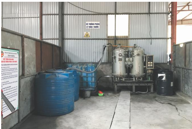
Oil – water separation system
